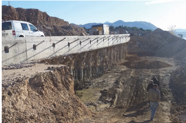
Fig. 6: Constructed anchored pile wall (bottom retaining structure)
